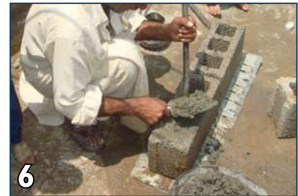
6 Repeat the procedure for filling all cavities..
