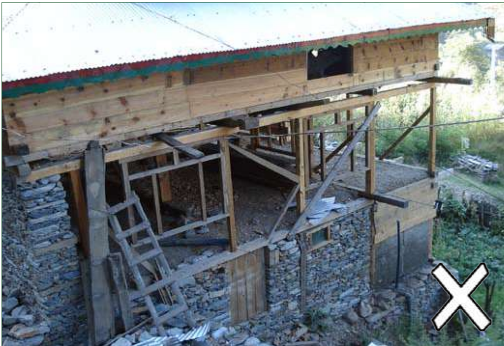
More than 1 storey retaining wall. Plan area not same for each storey.
