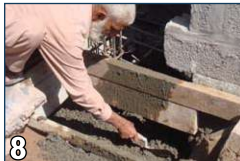
8 Pour 1:2:4 concrete in the foundation trench and the plinth band/beam
