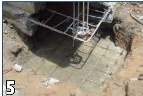
5 Clean the surface of the P.C.C. and place #3 bars @ 8" spacing on both ways in the form of mesh over P.C.C. surface
