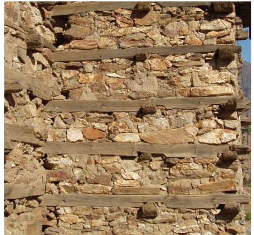
Traditional Bhatar construction Besham Fort (c. 1750) NWFP - Pakistan
