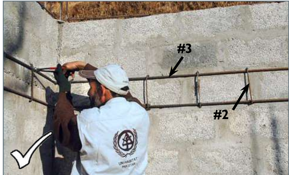
Method- 2: Widen the lintel and roof bands up to 10" For further details see Compliance Catalogue Section D (Remedial Measure)
