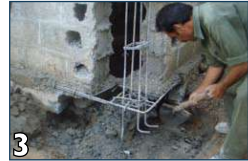
3 Chisel the existing plinth beam/band without destroying the existing reinforcement
