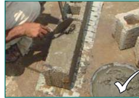
Fill hollow blocks to make solid wall
