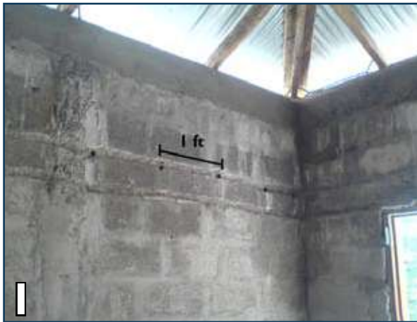
1 Clean the surface and drill holes.
