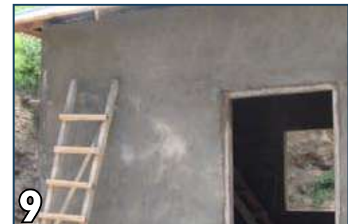
9 Cure the plaster at least for 10 days.
