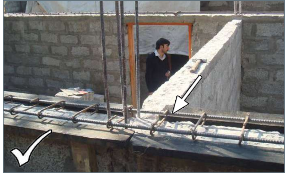
Method- 2: Widen the lintel and roof bands up to 10" For further details see Compliance Catalogue Section D (Remedial Measure)
