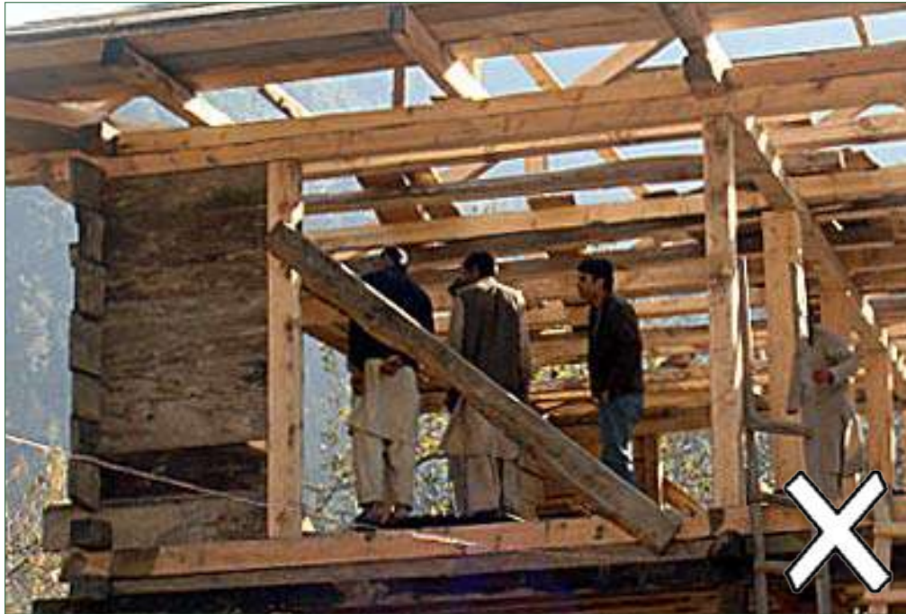
Distance from the corner to opening must be minimum 5 ft.
