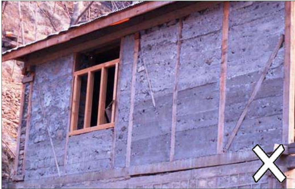
In situ concrete infill.
