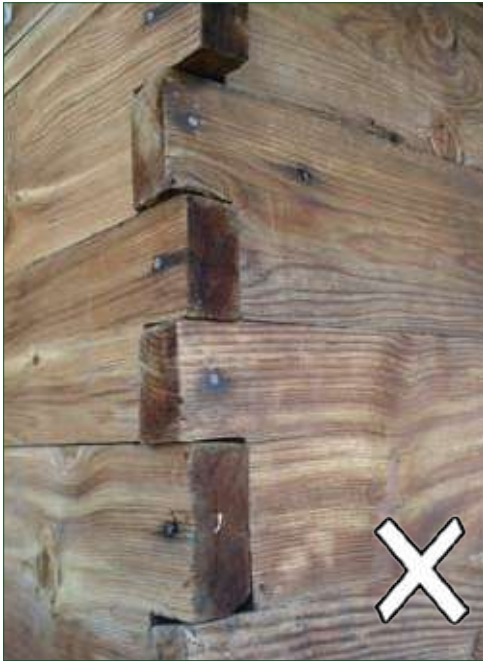
Boards ends not protected, nailed at weak location.
