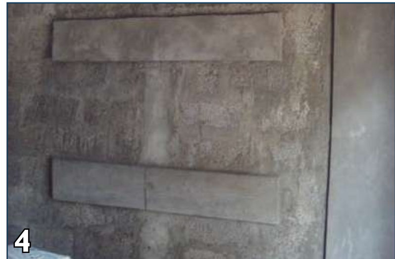
4 After final layer of plaster cure it for at least 10 days.
