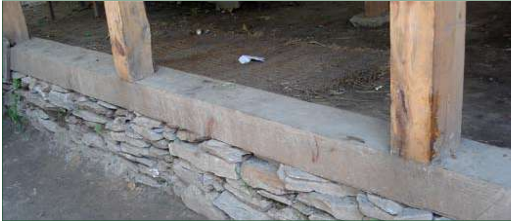
A good plinth protects the base plate and ensures it dries quickly.
