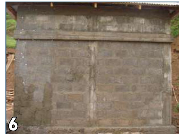
6 Cure concrete for at least 10 days.
