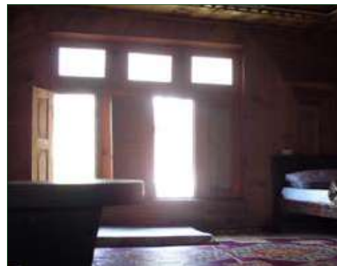
Large window frames should have sub frames like this.
