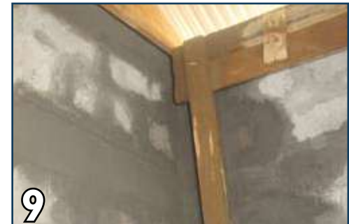
9 Cure the concrete for at least 10 days.
