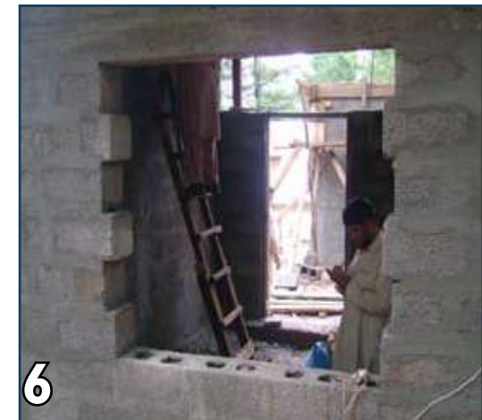
Tootthing left for providing the RCC frame around the opening.
