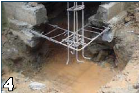
4 Dismantle the foundation 18" on both sides of the column
