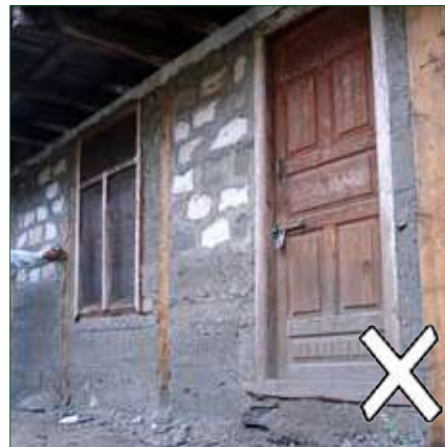
Masonry with sand cement mortar.
