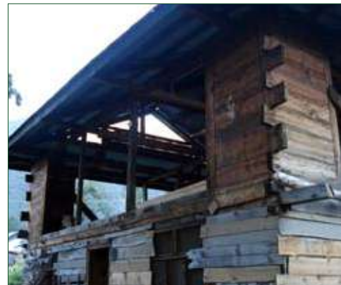
Thin boards may split or warp, nailed at weak location.
