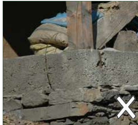
RCC beam has no connection to the timber posts. The frame is not well connected. Framing must be all timber
