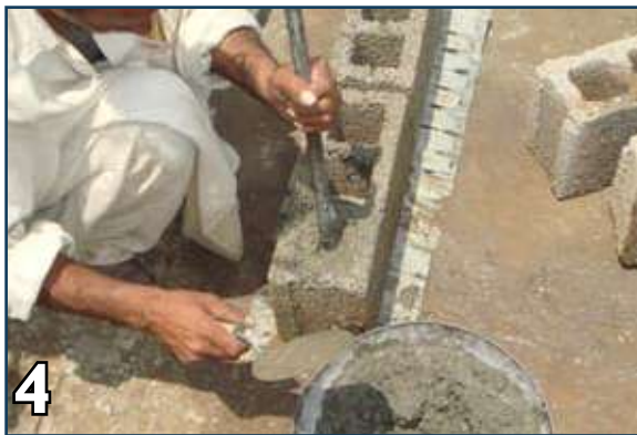
4 Compact concrete in layers with rodding.
