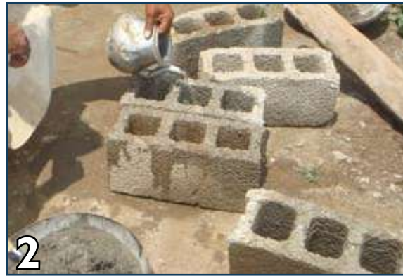
2 Wet the internal surfaces of the cavities in the blocks.
