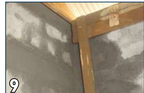
9 Cure the concrete for at least 10 days.
