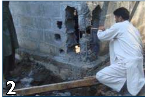
2 Remove the masonry in tooting pattern
