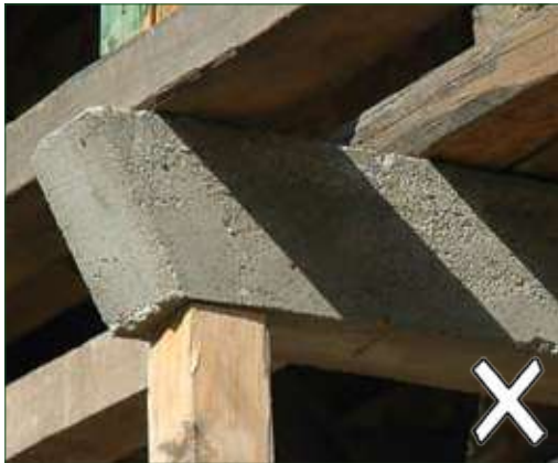
RCC beam has no connection to the timber posts. The frame is not well connected. Framing must be all timber
