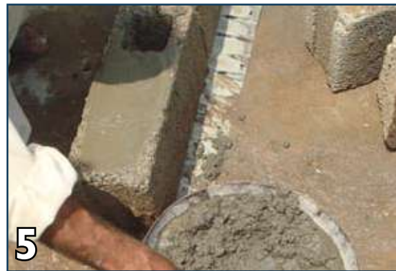
5 Level the surface after roding.
