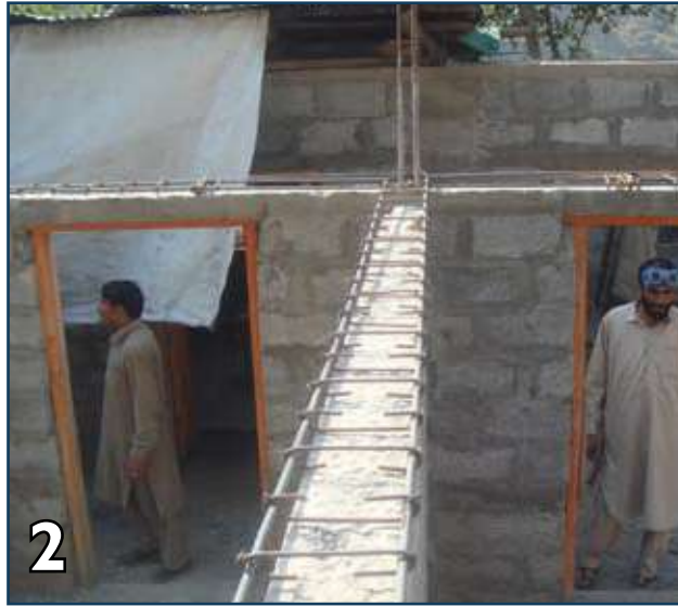
2 Fix 2- #4 longitudinal bars with #2 stirrups @ 6" spacings.
