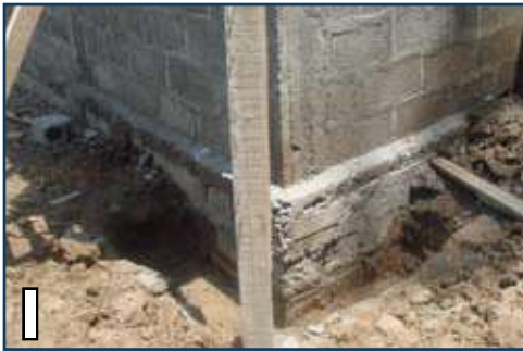
1 Prop the roof properly and dismantle the foundation in arch
