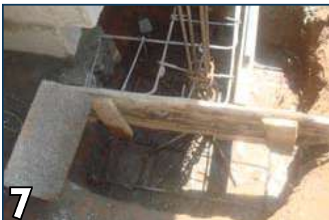
7 Place shuttering for plinth for pouring concrete
