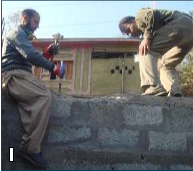
1 Dismantle the masonry above the existing lintel band.
