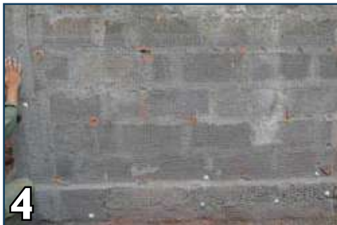
4 Place the wire mesh on both sides of the wall.
