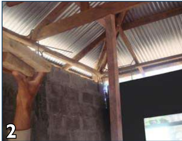
2 Support the roof with wooden props.
