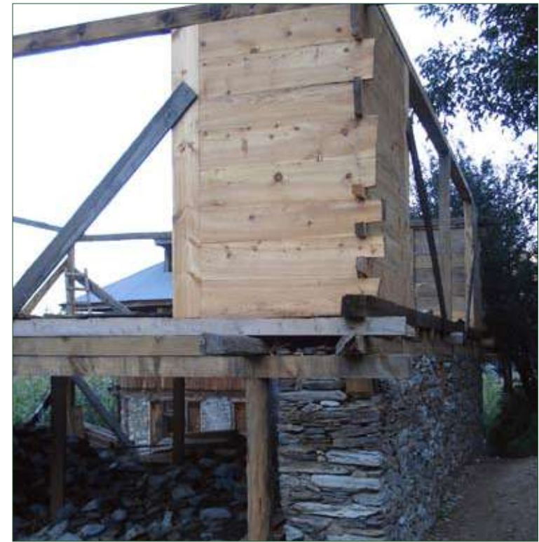
Upper storey frame is fixed to top of the wall.
