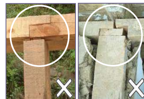
Do not put a joint directly over a post..
