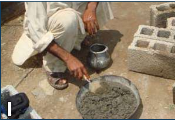
1 Mix 1:3:6 (cement:sand:aggregate) for filling the blocks.
