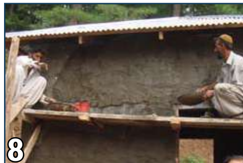
8 Apply 1" thick 1:4 (cement:sand) plaster on both faces of the wall.
