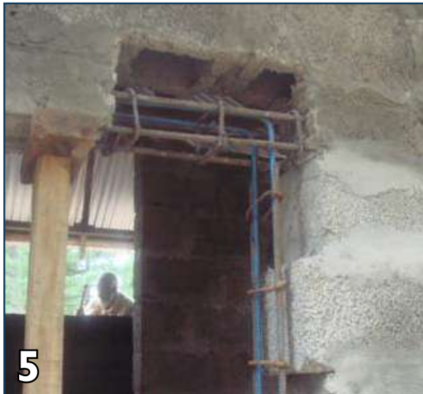
5 Reinforcement embedment in lintel beam/band.
