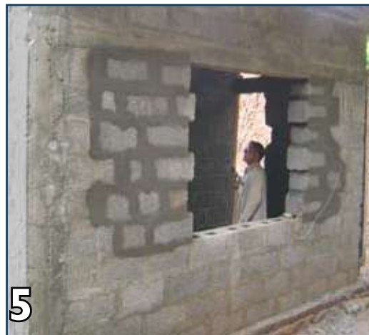
Opening size has been reduced and distance from center has been increased
