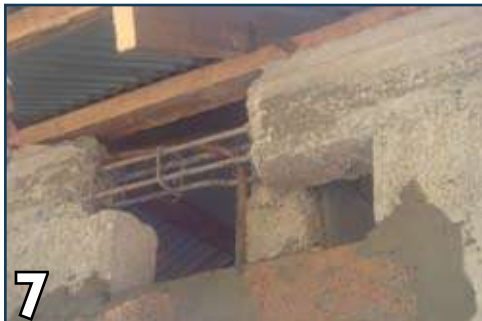
7 Embed vertical bars upto 8" in roof beam/band
