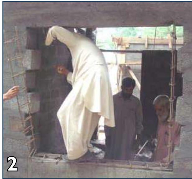
2 Place 2- #4 main bars with #2 @6" spacing stirrups.
