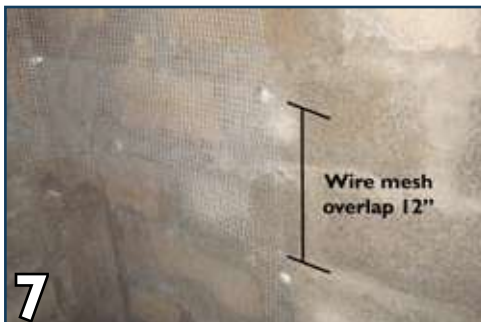
7 Provide min. 12" lap in wire mesh, where required.
