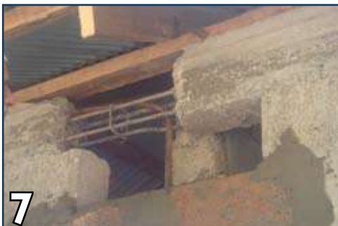
7 Embed vertical bars upto 8" in roof beam/band
