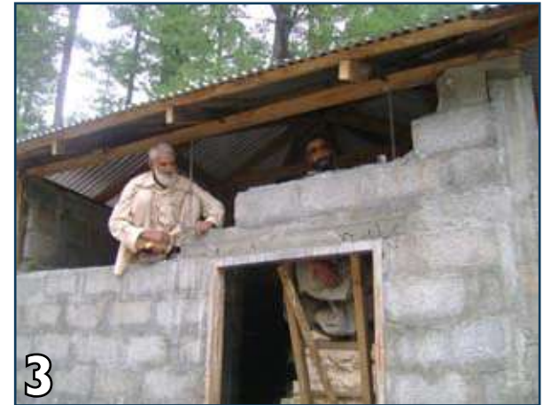
3 Remove masonry above lintel level and short lintel over the door.
