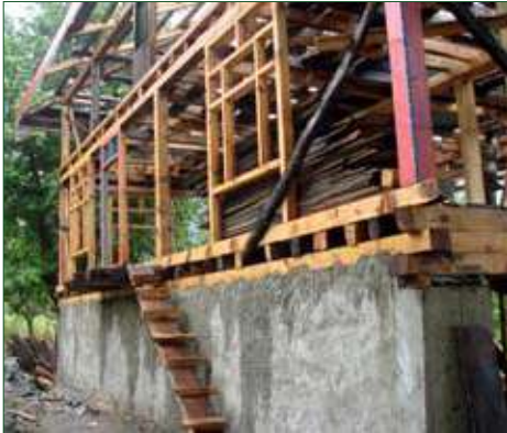
Traditional practice is to have back wall of stone.
