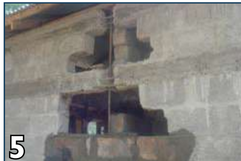
5 Ensure vertical bar passes through lintel band.
