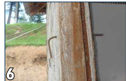
6 Fix 1/8" dia. L-bar in the holes and turn the bar from other end in U-shape as shown in Step -3.
