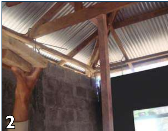
2 Support the roof with wooden props.
